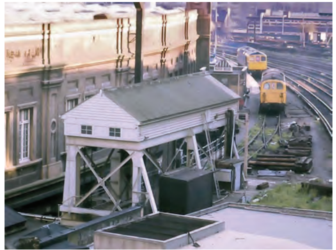
The WG Armstrong hydraulic lift in September 1974. Photo from KDH Archive
